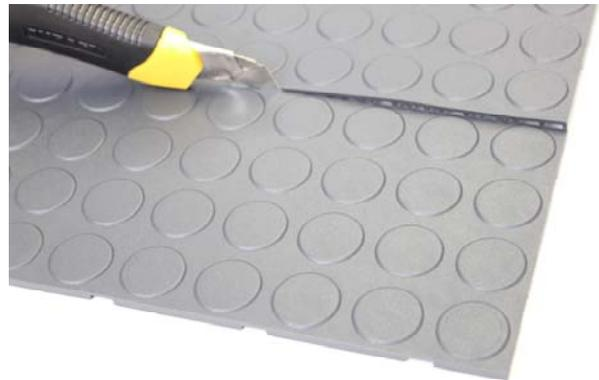
Take note of holes, posts, radiators etc.. Fit each mat into place and make necessary cuts with snap-off knife or secateurs.
