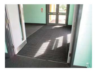
Combo 16 mm heel proof interlocking tile is fully compatible with the Integra 16 mm carpet tile.
