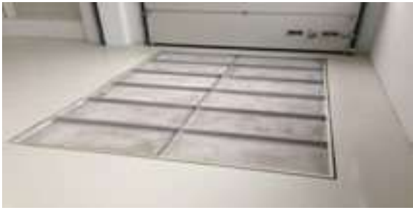
Example of MH 43 Hercules recess fabrication
